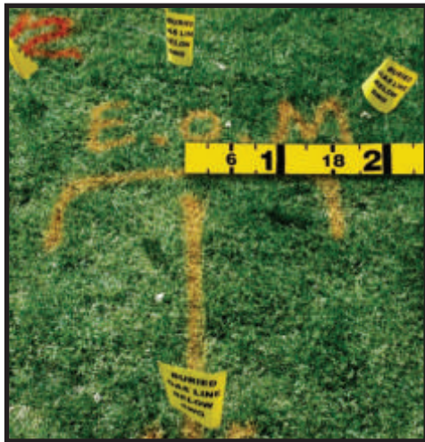
Document the markings before you dig
